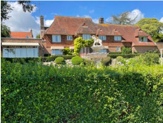
Rear elevation overlooking Clays Field
